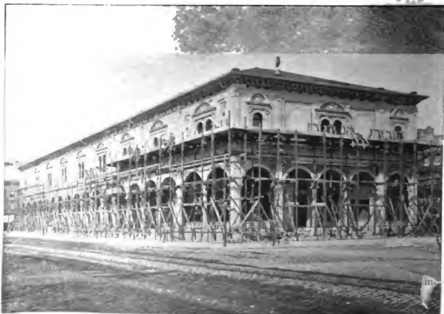
NEW-YORK HERALD BUILDING (IN CONSTRUCTION), BROADWAY AND 35TH STREET.
